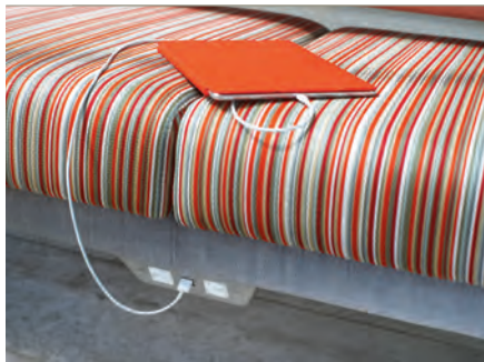
Under-seat power unit with custom housing features two outlets and two USB charging ports for maximum utility.
